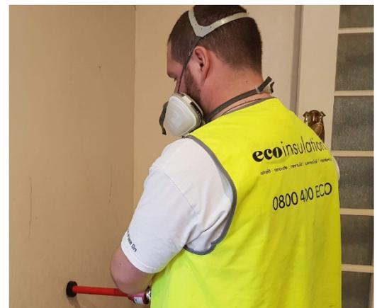
Installing insulation into existing houses improves the thermal performance of that building. The installation of Supafil® Frame dry glasswool into the external wall cavities reduces the loss of heat during winter, and overheating during summer. Wall insulation saves money by reducing your heating costs. Supafil® Frame is non-combustible, with high R-values (where installed) in comparison to other exterior wall insulation types.
